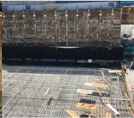
E.Proformance Shoring applied over geofoam blocks with horizontal penetrations and tie-backs
