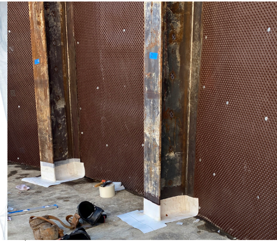
Field fabricated pile detail boots.
