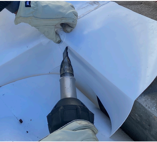
Heat weld detailing an inside corner at an elevator pit.
