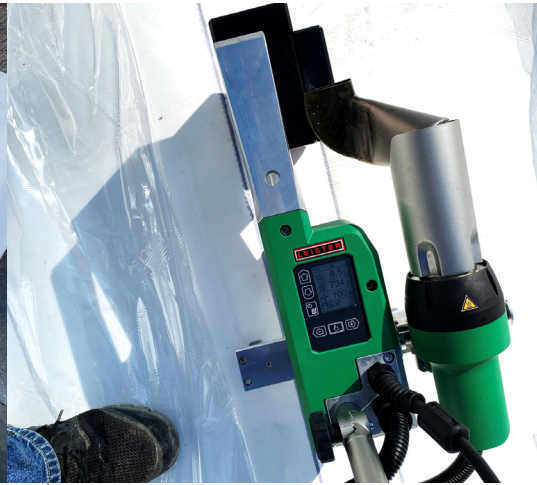
Horizontal heat weld with welding equipment.
