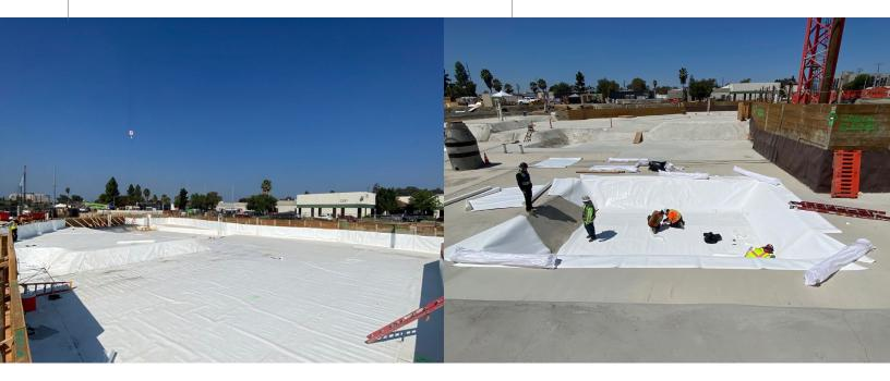
approximately 230,000 square feet to form an underslab and blindside waterproofing and methane barrier.
