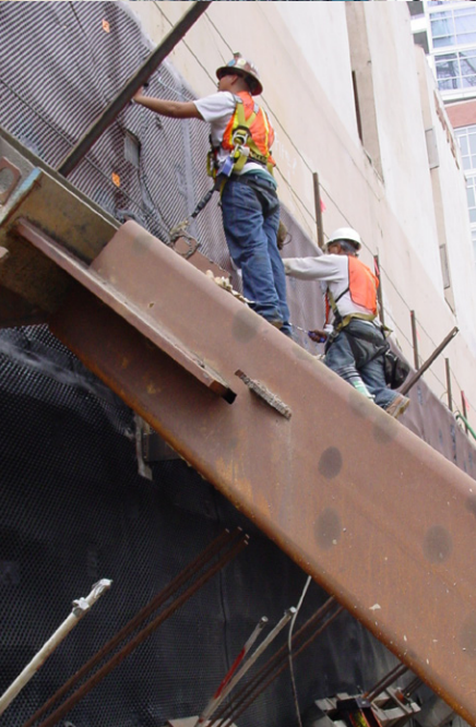
Waterproofing crews providing detailing around rakers near the top of grade.
