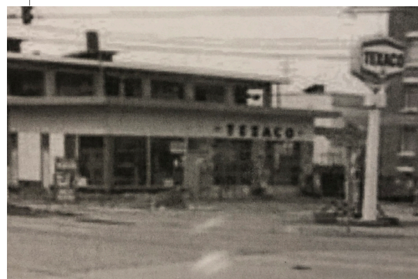
Original Texaco station that operated on site for 70 years from 1923 - 1993.
