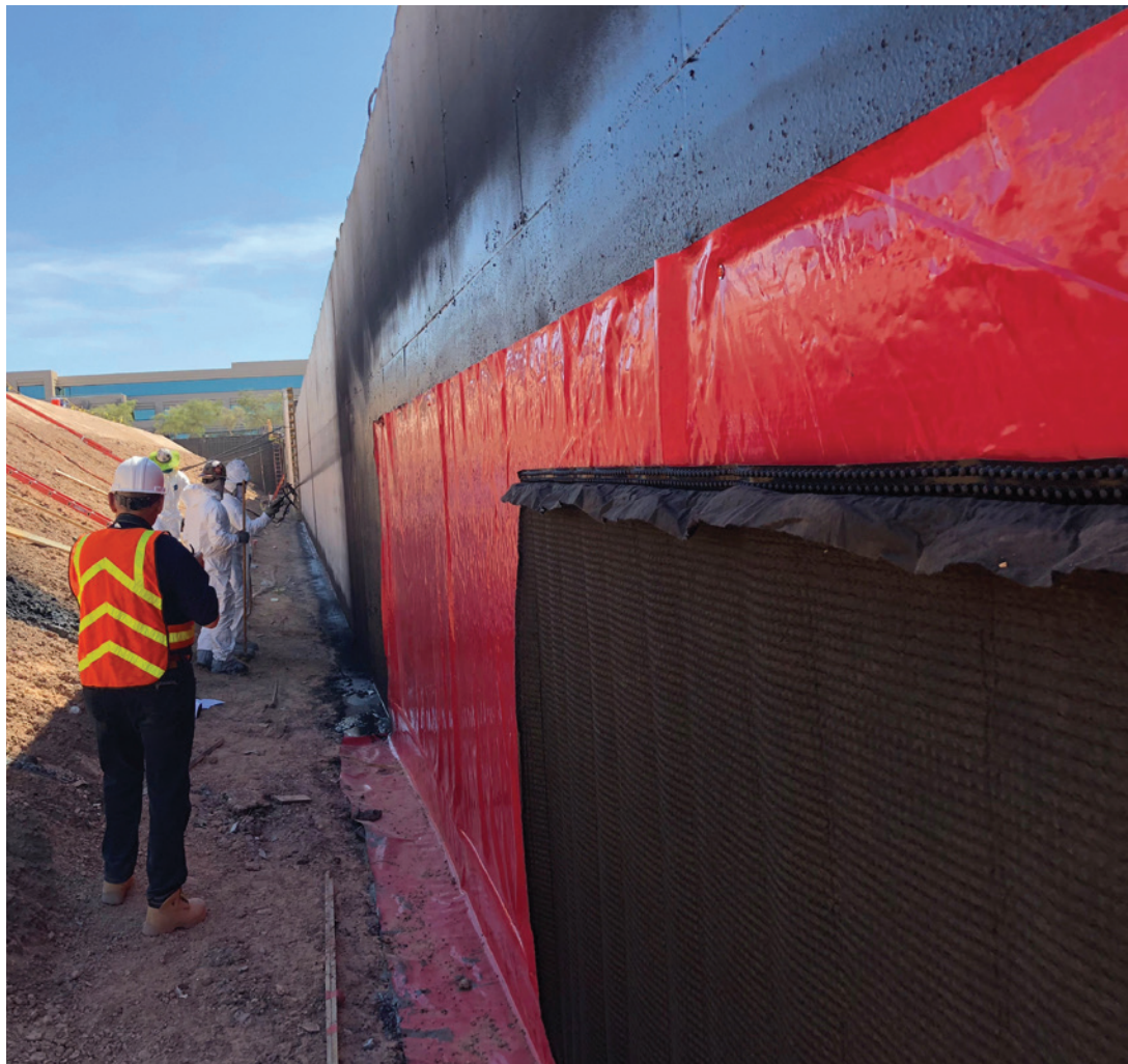
E.Protect Wall System assembly: e.spray 80 mil, e.shield 115, and e.drain 6000
