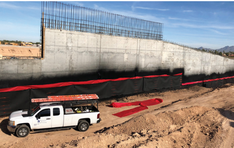
Application of E.Protect at first lift.
