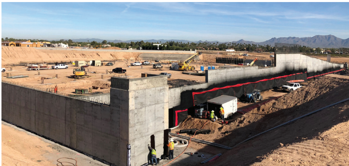
Application of E.Protect at first lift.
