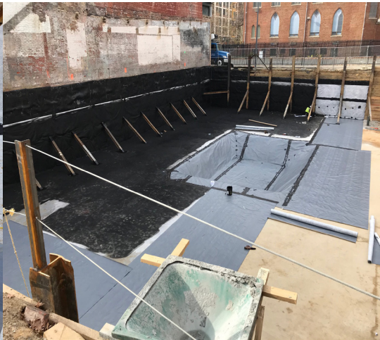
Installation of e.base 205 and e.spray on underslab and below grade walls.
