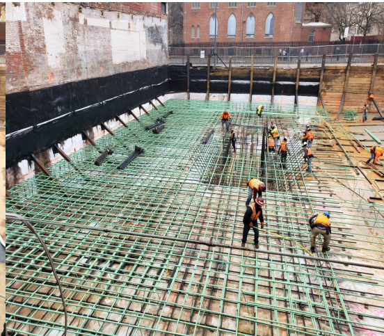
Rebar installation after system installation is complete.
