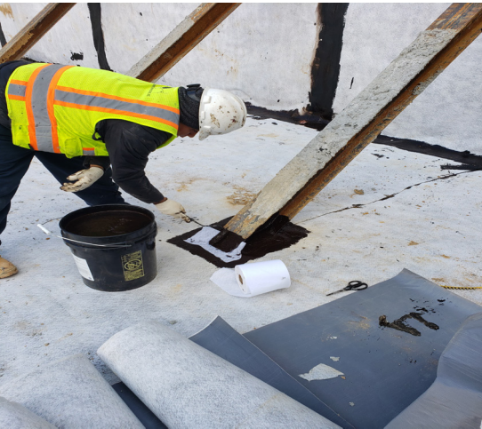
Hand detailing around raker.
