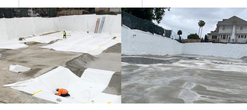
It is comprised of the PreTak membrane, a high-density polyethylene (HDPE) sheet that once installed provides a tough and durable chemical resistant waterproofing, methane, and contaminated soils barrier membrane.
